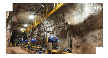
B Underground Pump Station – prep and install concrete, steel and formwork. Install all suction and discharging pipe work. Intall monorail and main water storage hopper. Install 5 x WT088 pumps and commission
