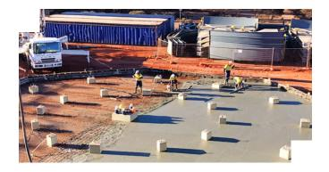
Crusher Plant - complete all civil & trenching works required for new crusher and screening. Concrete to AS3600, all excavation, steel fixing, formwork by Rangecon. 6 Degrussa Mill Upgrade – complete concrete and civil works to new thickener and filter building with suspended slab. Concrete to AS3600, all excavation, steel fixing, formwork by Rangecon.
