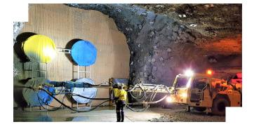
**10** Construction of ventilation walls and spray with shotcrete. Installation of ventilation control systems, such as pneumatic ventilation doors and DBR's.
